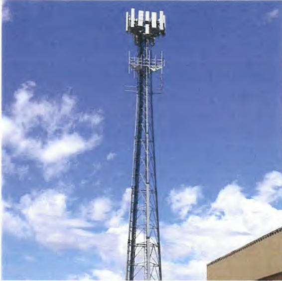
Communications tower - towers are all similar in appearance
