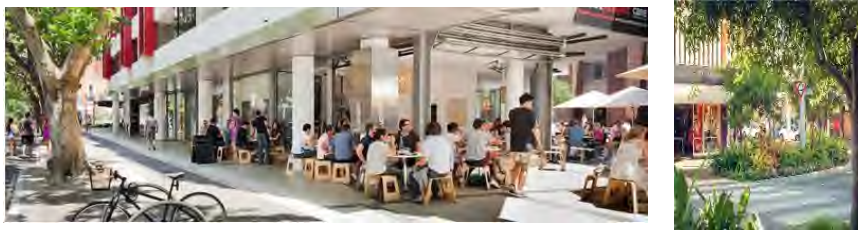
Figure 17: Examples of an actively engaging development, with mixed uses on the ground floor
