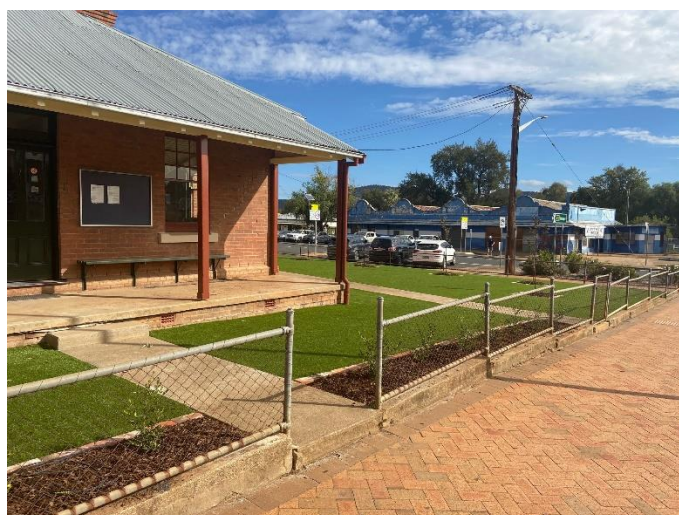
Figure 2: New front landscaping of the Old Wellington Police Station
