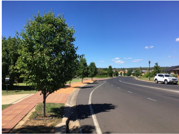
Photograph 4: St Andrews Drive following replacement. Age of trees approximately 5 years (2017)
