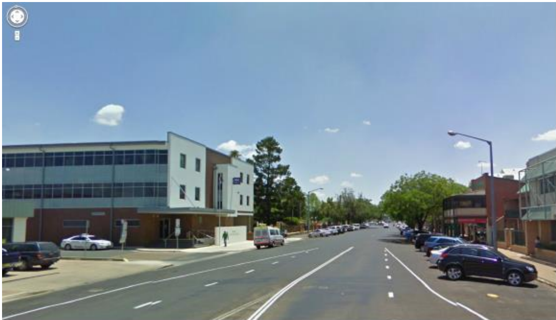
Figure 3: Brisbane Street prior to the Stormwater Augmentation Civil Works
