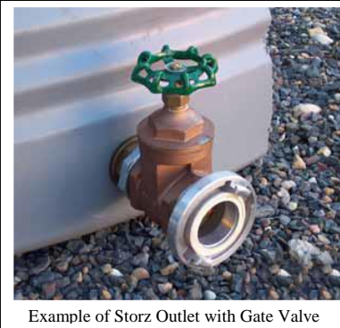
Example of Storz Outlet with Gate Valve
