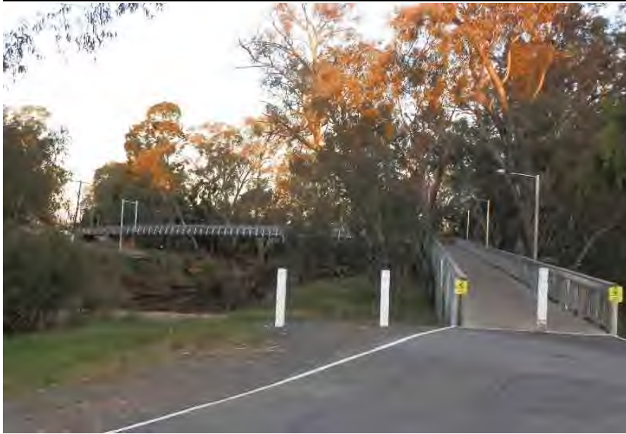
Campaspe River Footbridges, Echuca
