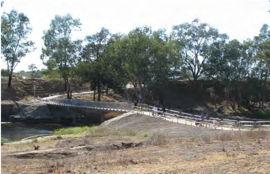
The unsuitable Dubbo Tamworth Street truss footbridge (causes major log jams in floods and impacts on river flow, causing major erosion and change to river flow and lacks character and visual appeal and heritage-historic-style of Wellington.
