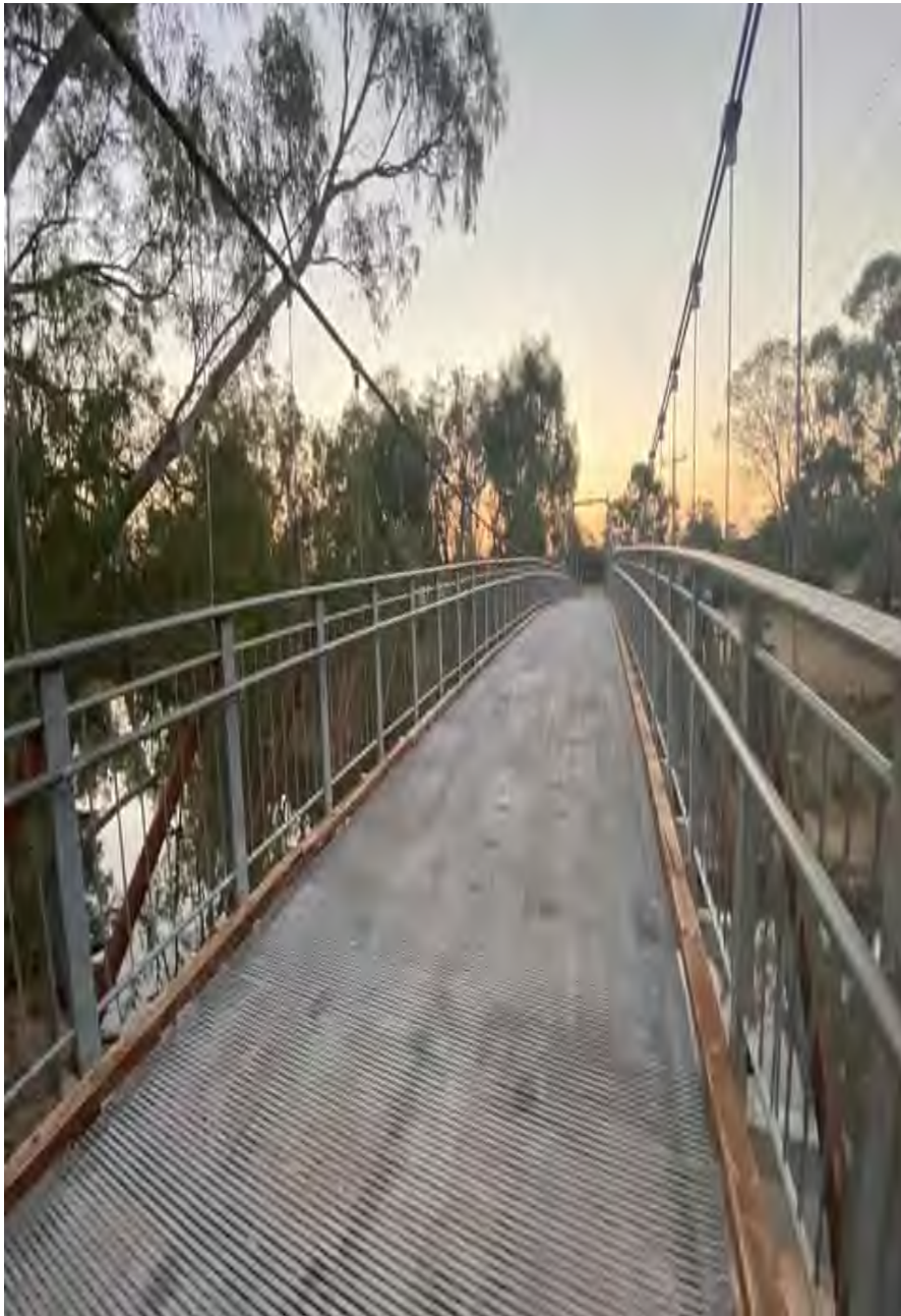
Campaspe River Footbridges, Echuca
