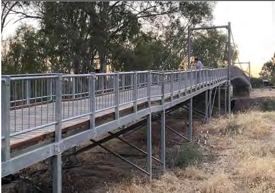
Campaspe River Footbridge, Echuca
