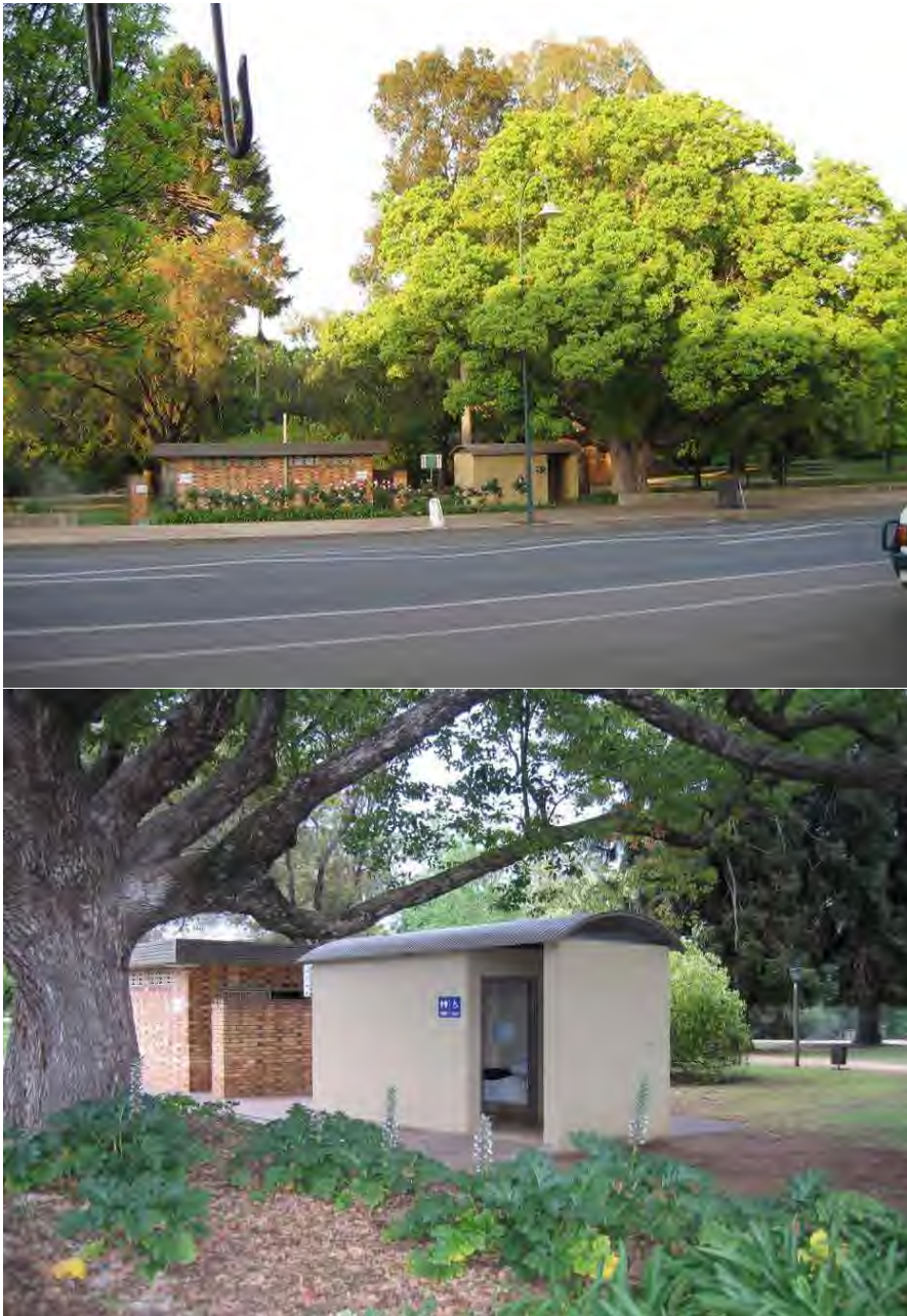
PHOTO: THE ORIGINAL CAMERON PARK AMENITIES BLOCK AND DISABLED TOILETS WHICH HAVE BEEN REMOVED AND REPLACED
