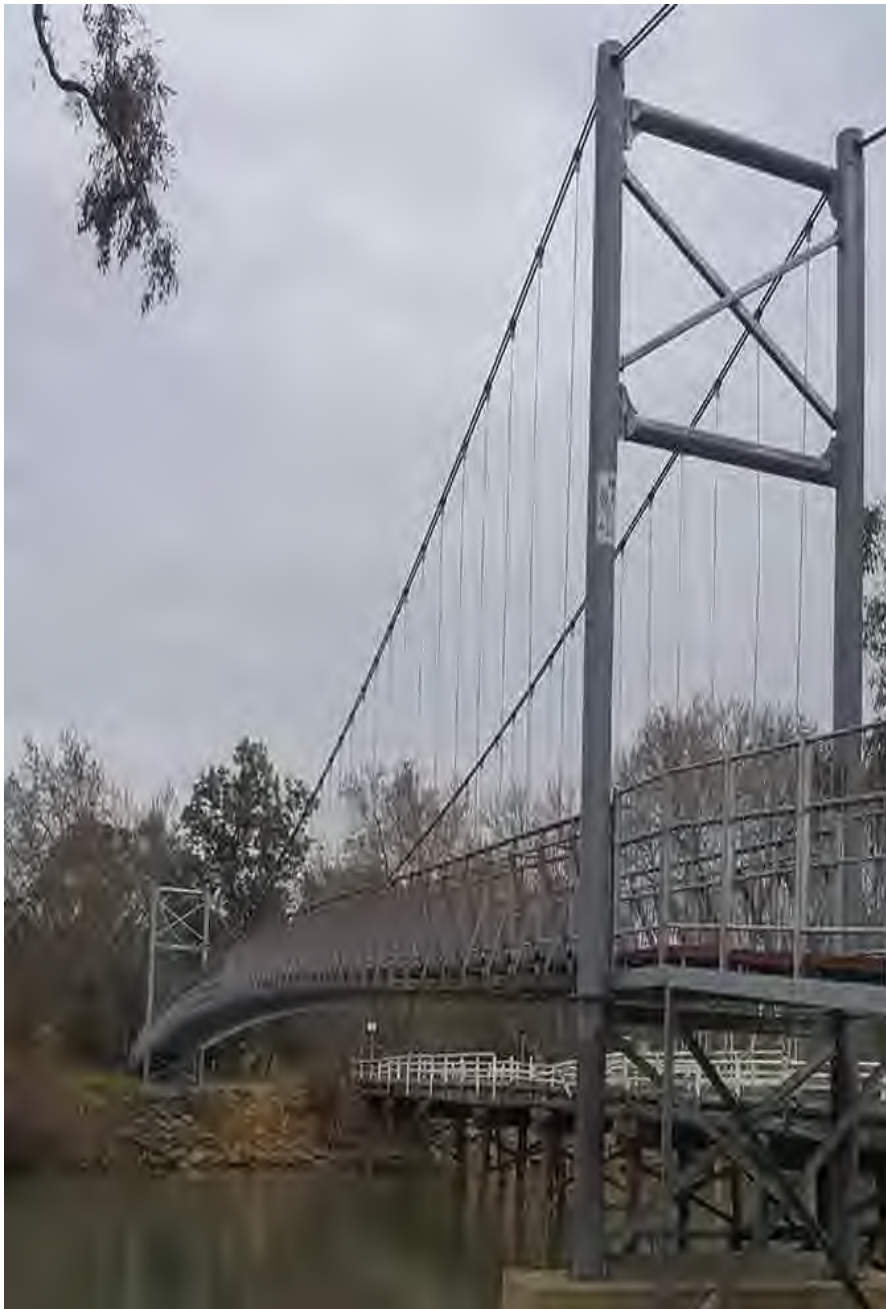
Moodie: Cable Bridges
