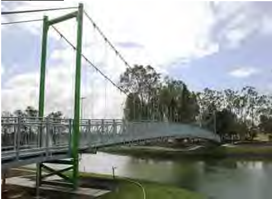
Rockhampton cable bridge (by Moodie) bridge.
