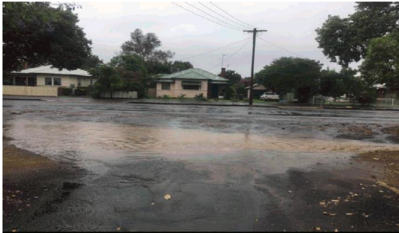
Photograph 2: View facing north from lane to the Bultje Street showing flooding. (2/12/2017)
