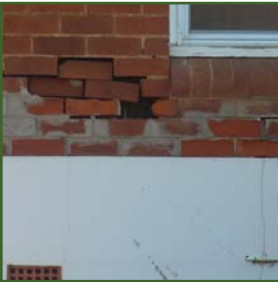
↑ Home and office buildings with salinity damage in South and Central Dubbo
