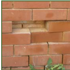
↑ Home and office buildings with salinity damage in South and Central Dubbo
