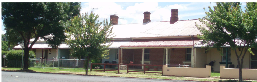
Figure 16: Row of terrace houses, Percy Street Wellington (Source: Strong, 2010).
