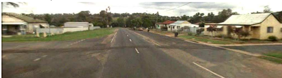
Figure 10: Intersection of Reid and Thornton Streets (Collector Streets) Wellington (Source: Google Maps 2010).
