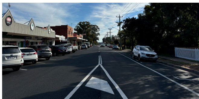
Tamworth Street reconstruction completed.
