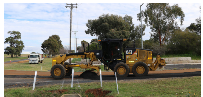
Ongoing road repairs.
