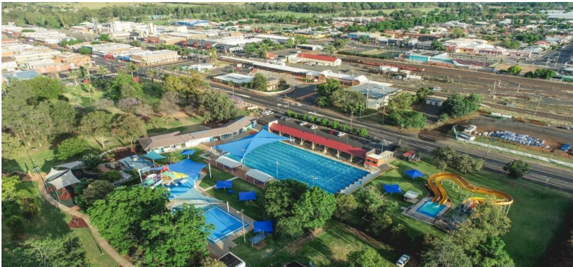
Figure 3 – Existing Dubbo Aquatic Leisure Centre
