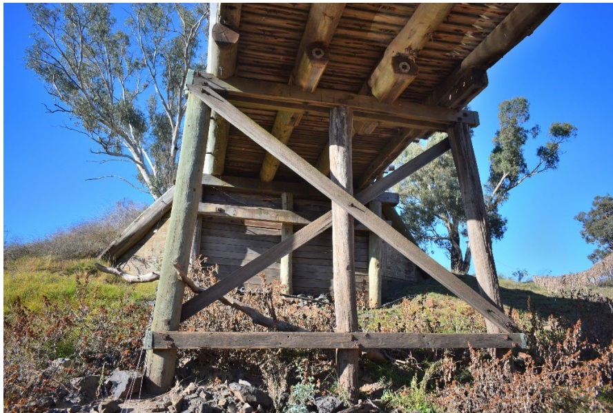
Figure 3-12 Typical trestle support (Source: FBE)
