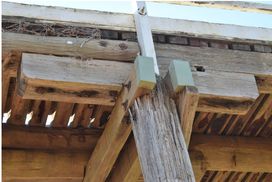
Figure 3-1 Old (original) square corbel element (Source: FBE)
