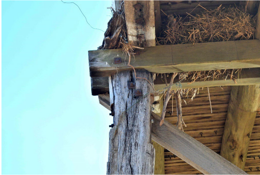
Figure 3-15 Splitting of the pile (Source: FBE)
