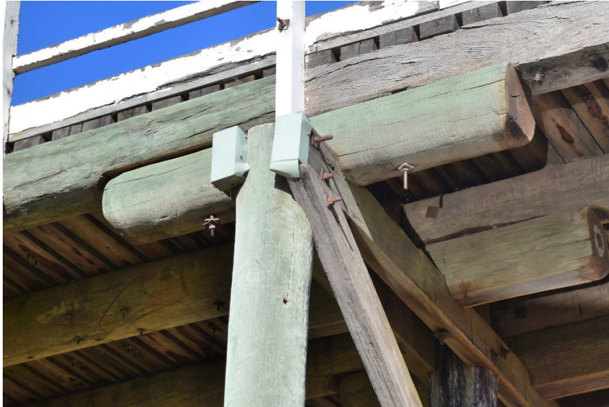
Figure 3-2 New corbel element (Source: FBE)
