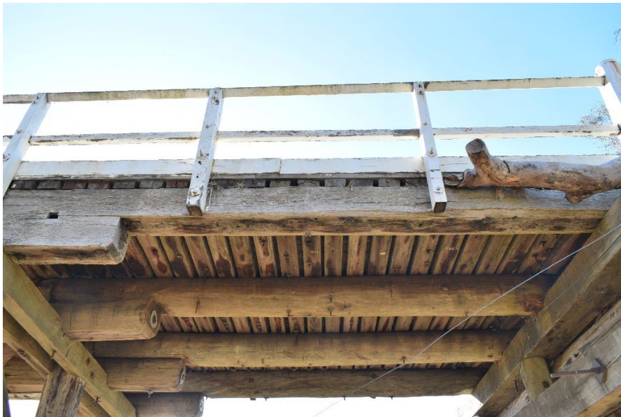
Figure 3-3 New and old girders at Span 4 (Source: FBE)
