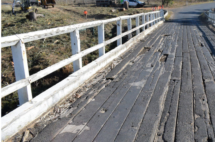
Figure 3-4 Typical barrier and kerb (Source: FBE)
