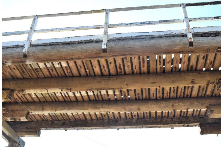
Figure 3-8 Superstructure soffit, typical condition (Source: FBE)
