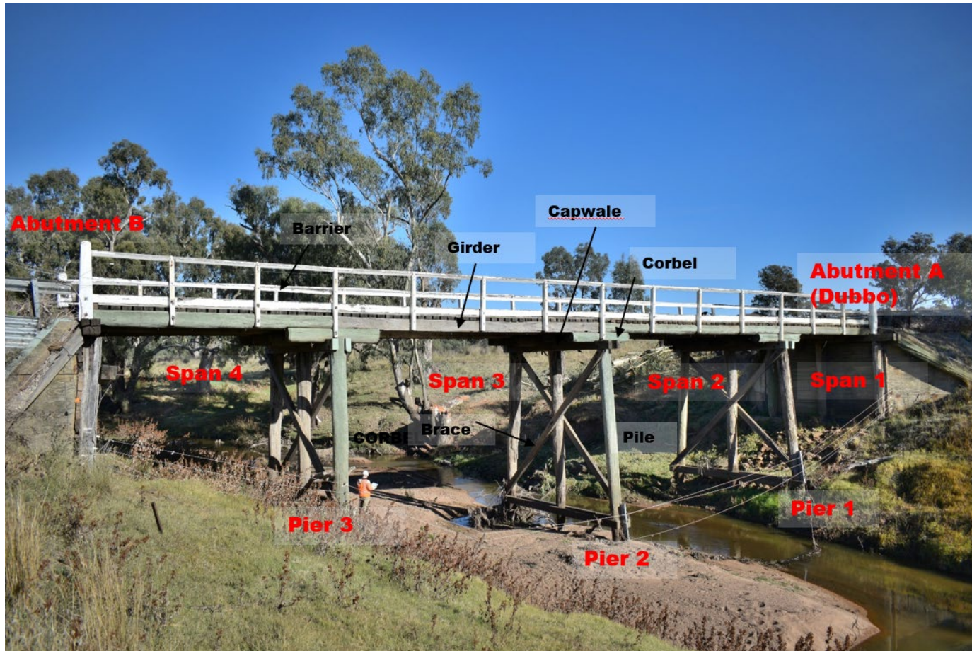
Figure 2-1 Benolong Bridge elevation (Source: FBE)
