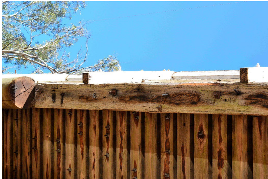
Figure 3-9 The old square section girder example, typical condition (Source: FBE)
