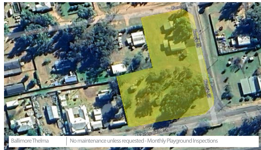
Ballimore Sporting Oval | No maintenance unless requested - Monthly Playground Inspections
