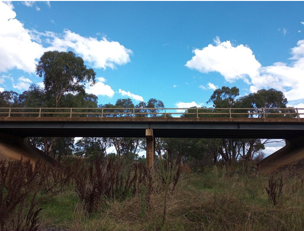
Figure D.1 Golden Highway Bridge on Ballimore Creek (view from downstream)
