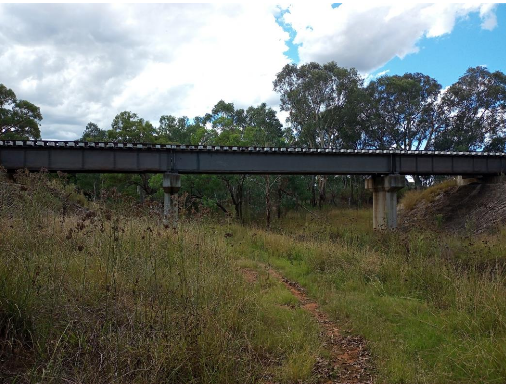
Figure D.2 Railway Bridge on Ballimore Creek (view from upstream)
