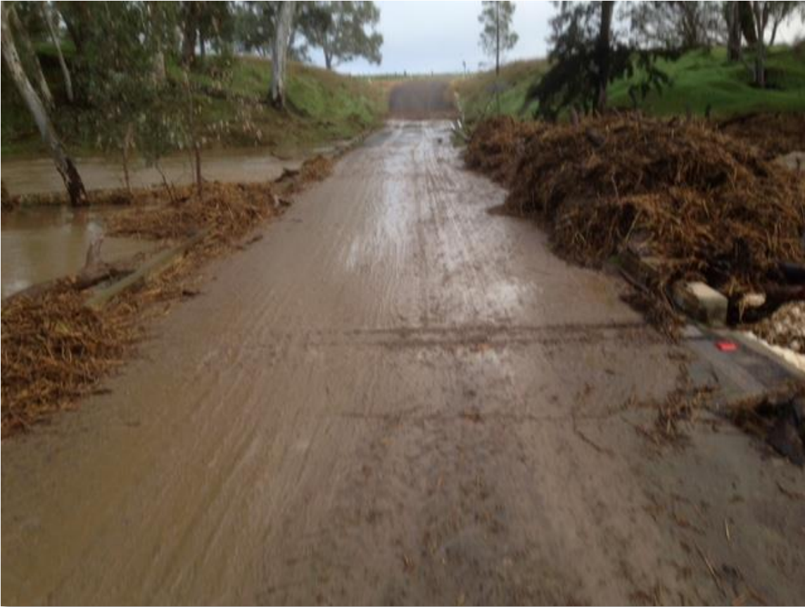
Figure 2.4 2010 Flood at Bill Mills Bridge (Source: Council)
