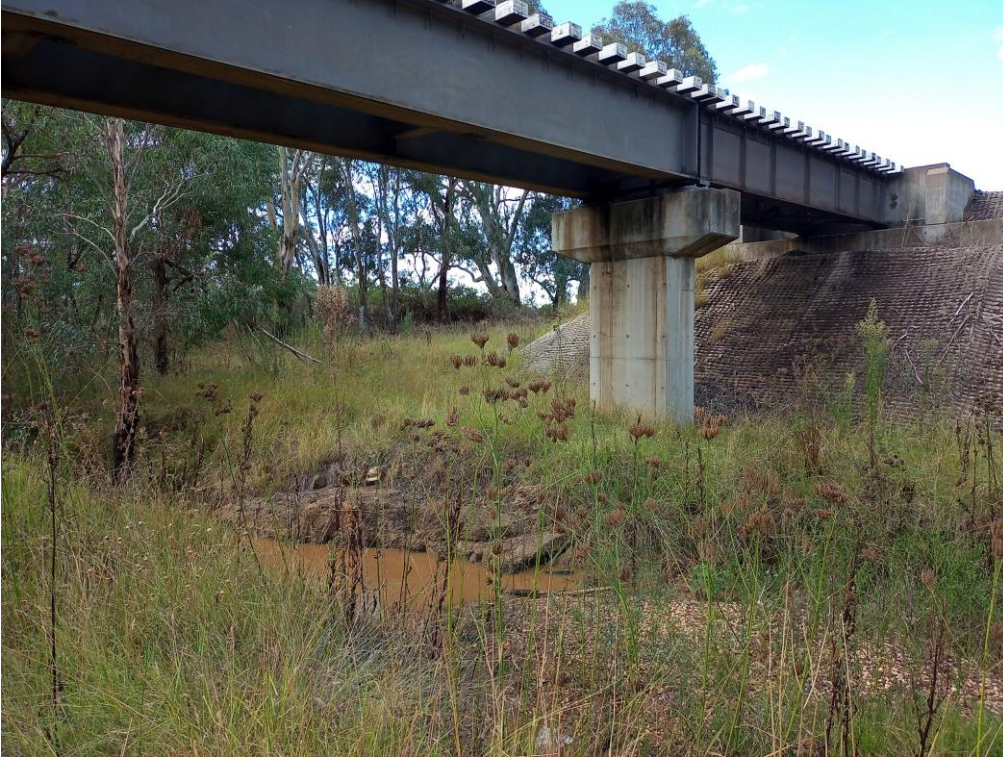
Figure D.3 Railway Bridge on Ballimore Creek (view from left bank)
