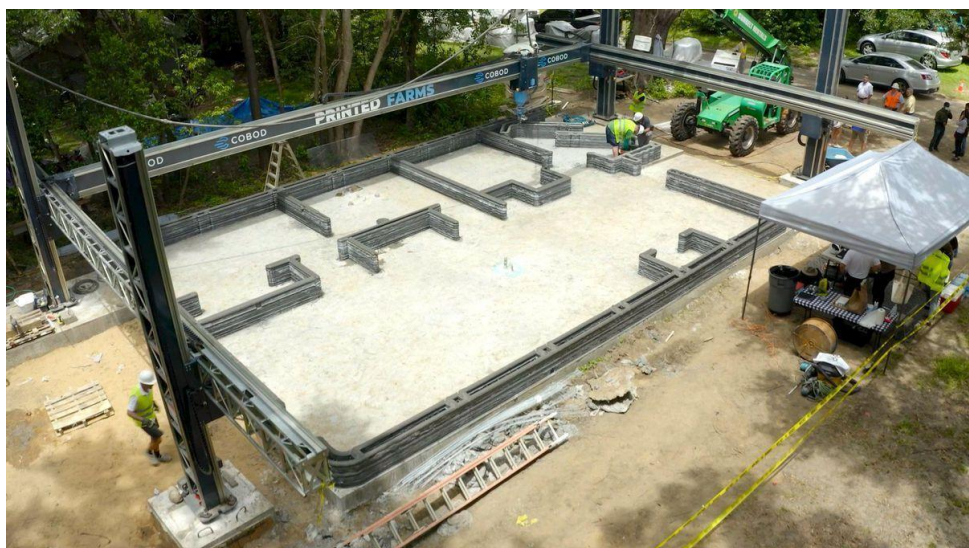
Figure 4 - Example of a gantry 3D printing system
