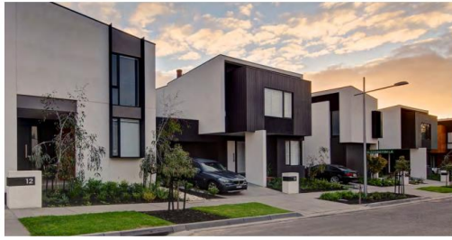
Figure 14: Low rise medium density housing with reduced setbacks and a range of design elements
