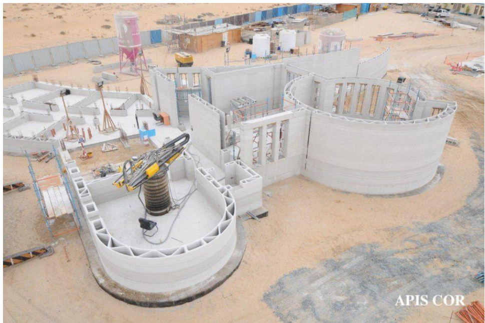
Figure 3 - Example of a robotic arm 3D printing system
