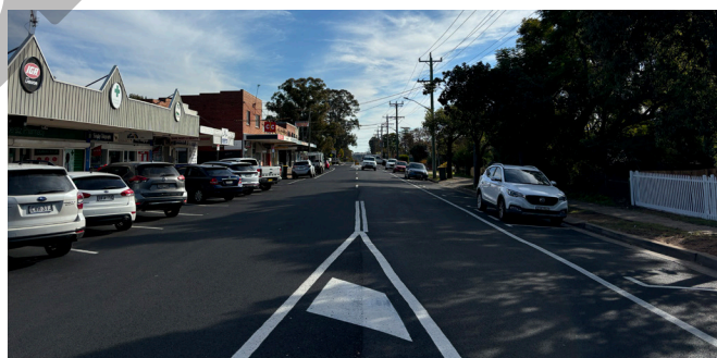
Tamworth Street reconstruction completed.
