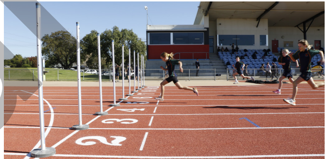
Barden Park resurfacing completed.
