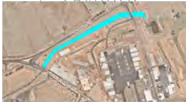
Figure 4: Open Stormwater Channel
