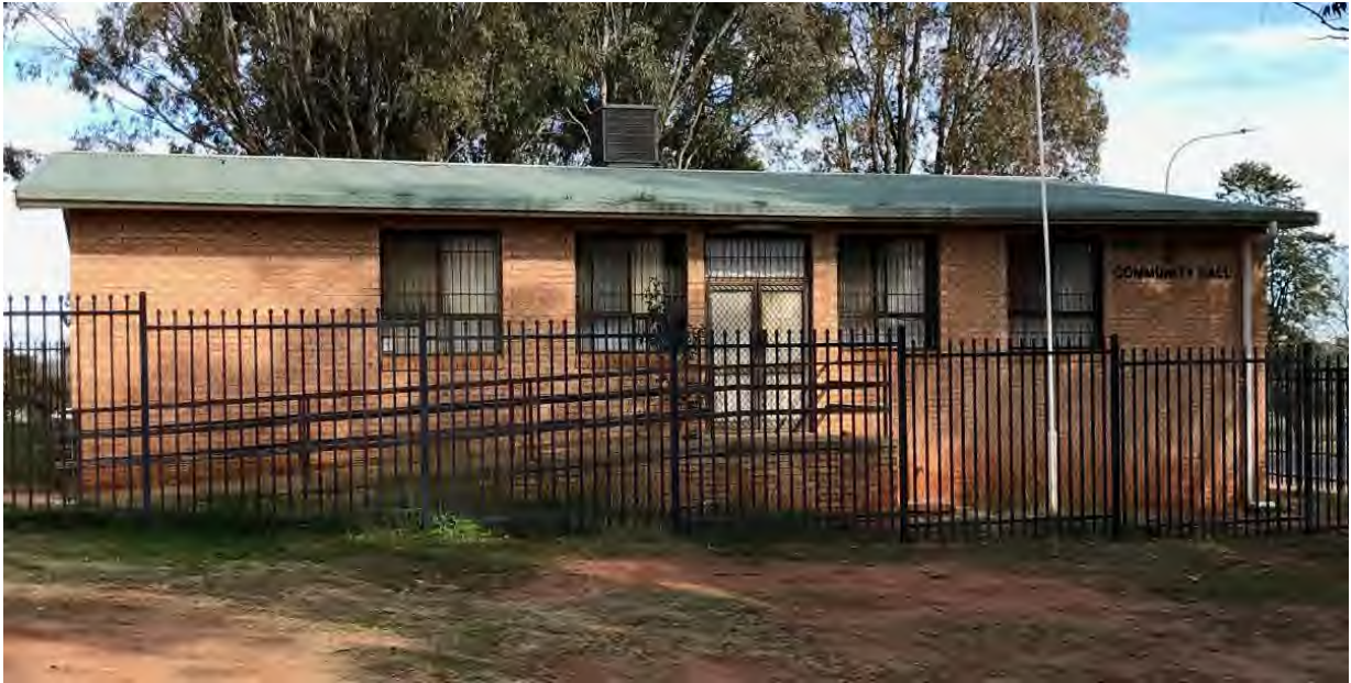
Figure 2. North facing entry to the building.
