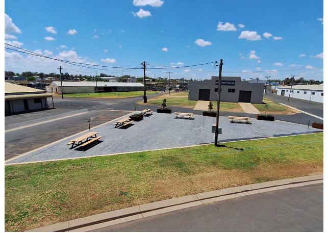
Dubbo Showground pavillion piazza
