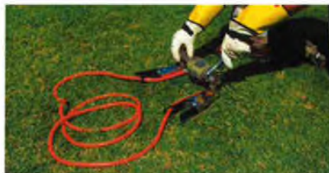
Bridging out of water meter
