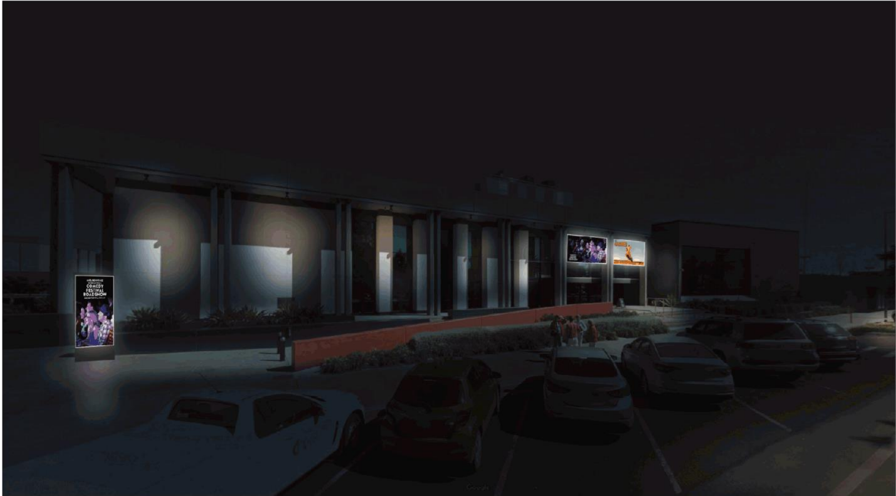
NORTHWEST FACADE VIEW
