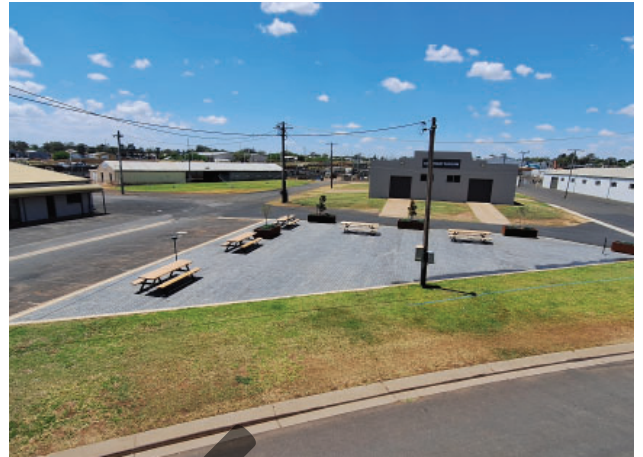
Dubbo Showground pavillion piazza
