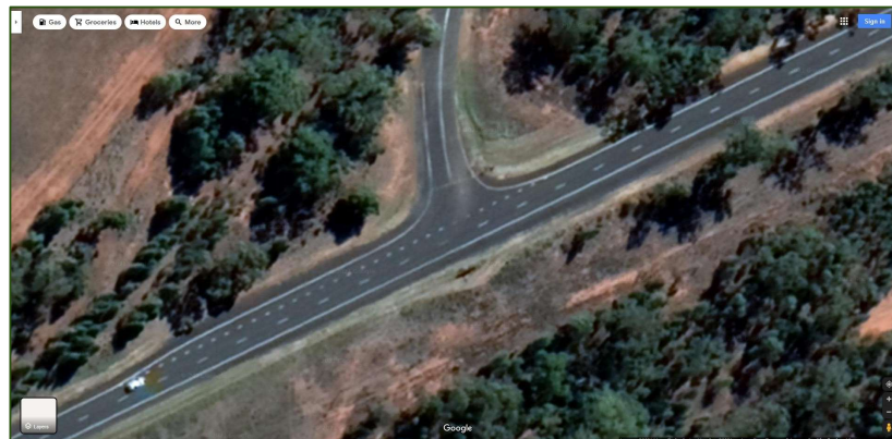
Figure 4. Google aerial photograph of the intersection, Old Mendooran Rd terminating at the Golden Hwy; Dubbo is to the west (left of photograph). Note the BAL and BAR layout.
