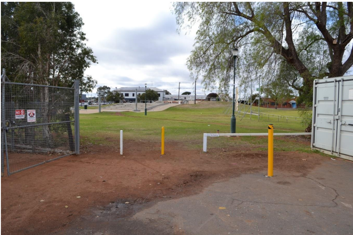
Figure 5: The replacement of rail fencing and boom gates with bollards, the yellow bollard being removable and therefore acting as a gate.
