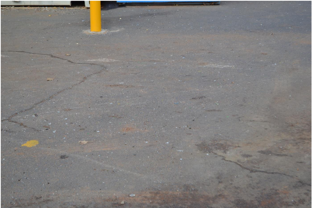
Figure 4: Small shards of glass left behind by the contractor emptying the reverse vending machine.
