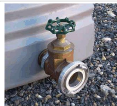
Example of Storz Outlet with Gate Valve
