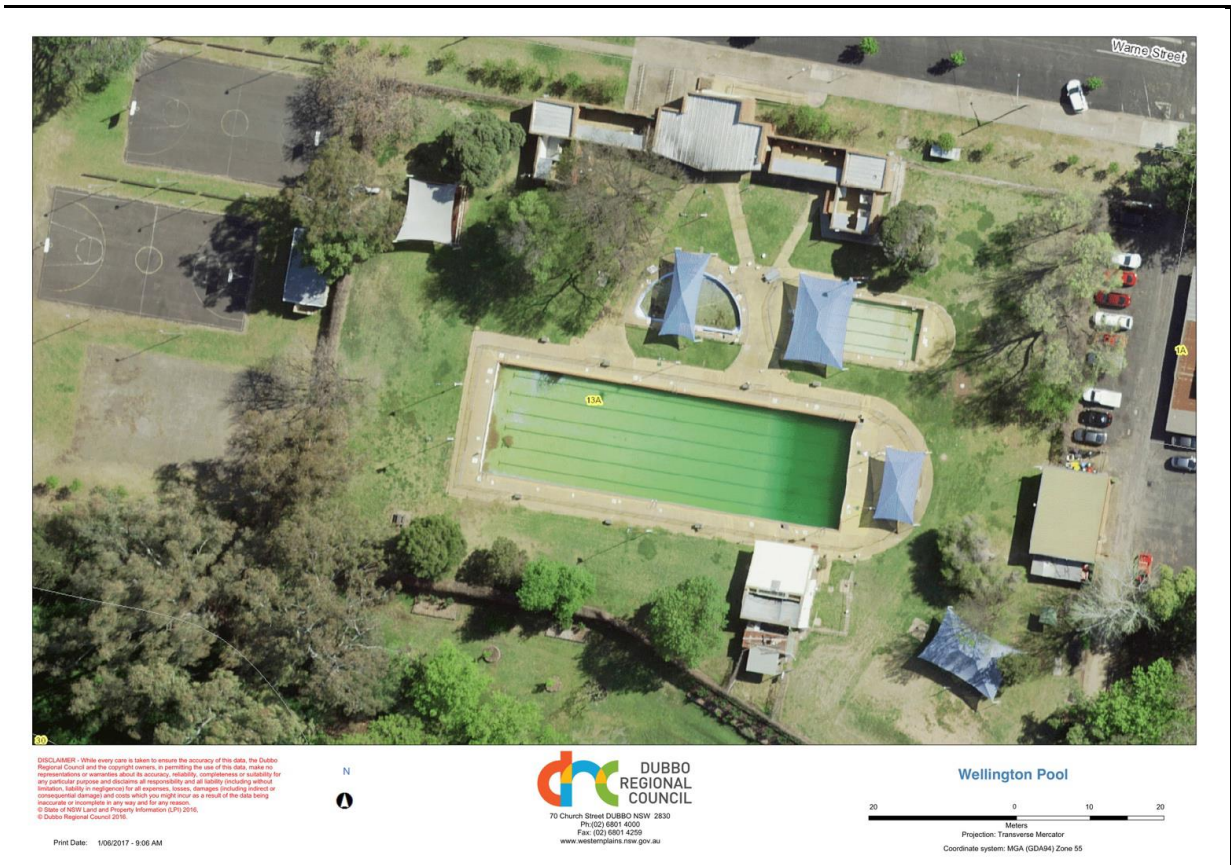
Figure 1. Wellington Pool Complex (current)
