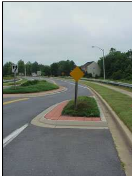
Picture 1 - Traffic calming devices
