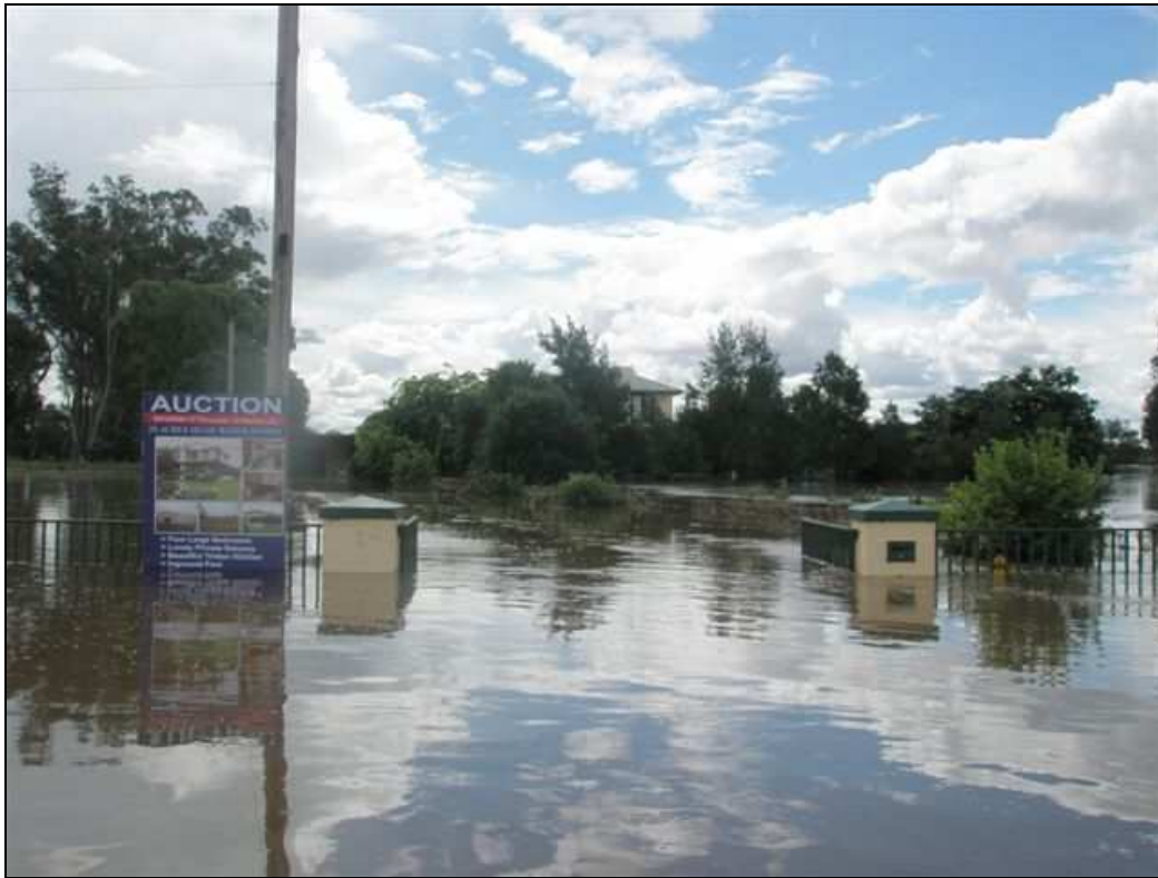
Photograph 6: Lack of flood-free access - December 2010
