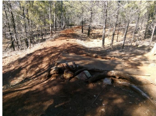
Photo 4-4: Rural levee to the south of Geurie
