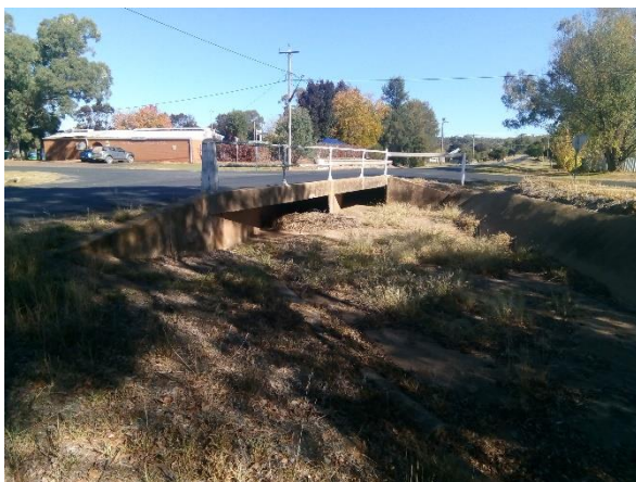
Photo 4-15: Mitchell St culvert over Boori Creek, looking south
