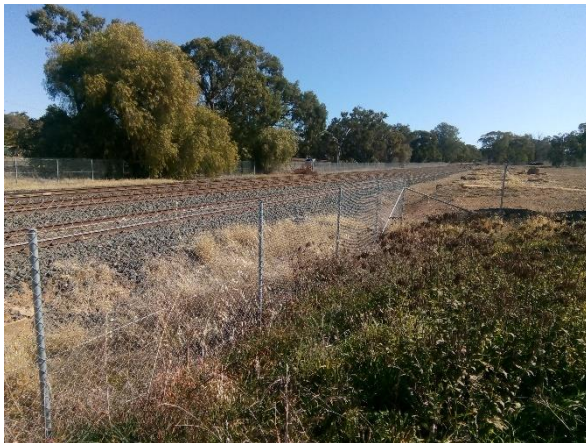
Photo 4-7: Railway embankment, north-side looking west
