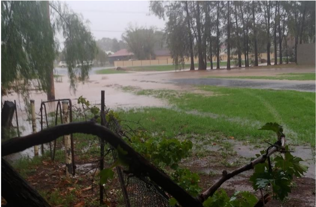
Photo 4-19: Boori Creek culvert across Jennings Street
