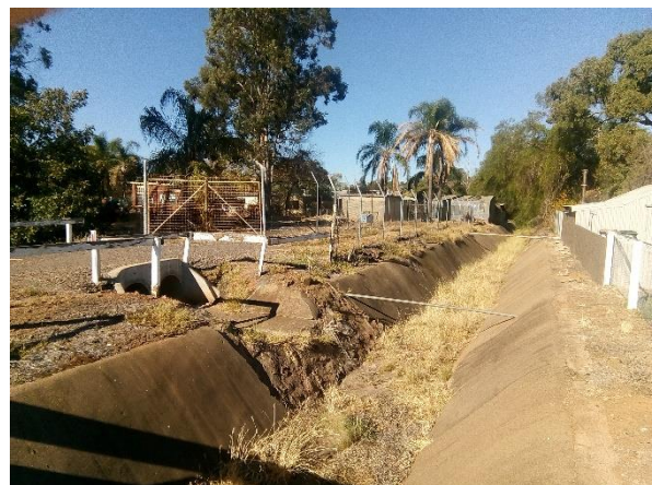
Photo 4-16: Boori Creek to the east of Chambers St
