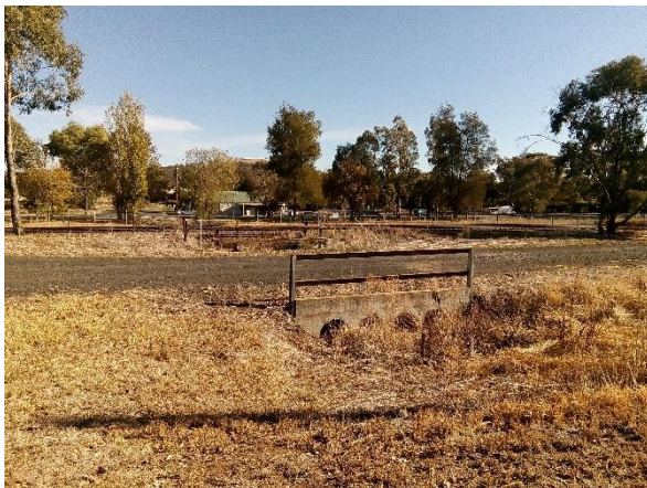
Photo 4-9: Culvert under Narragal St near the intersection with Chambers St
