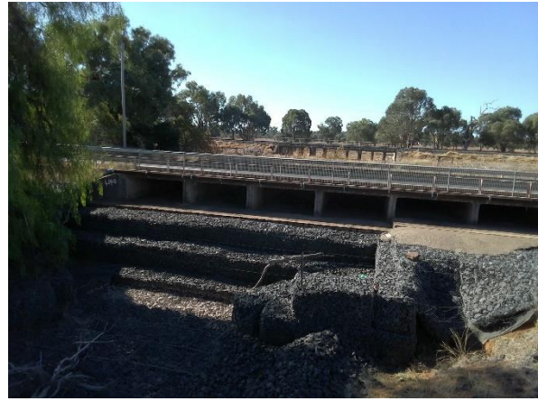
Photo 4-12: Mitchell Highway culverts over Geurie Creek, looking north
