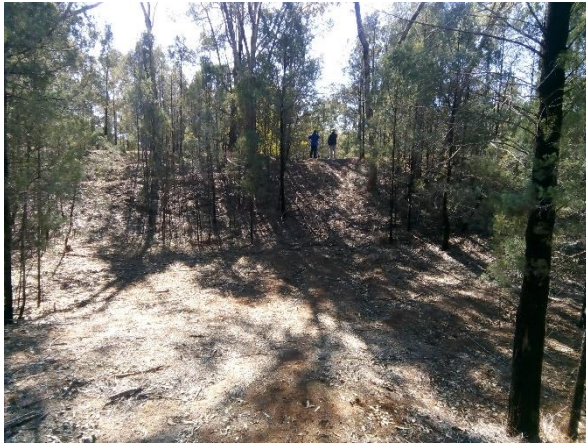
Photo 4-5: Detention basin to the south of Geurie
