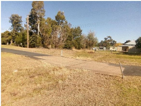
Photo 4-13: Jennings St Causeway over Boori Creek
