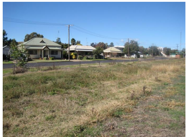
View east of houses adjacent to railway culvert
