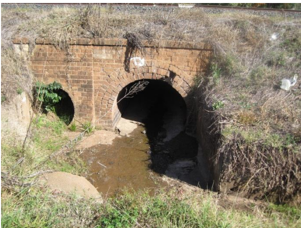
View downstream of railway culverts
