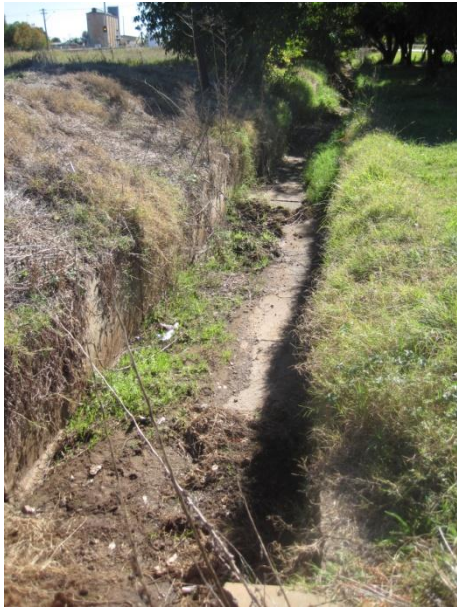
The overgrown concrete channel looking north upstream from the railway culvert
